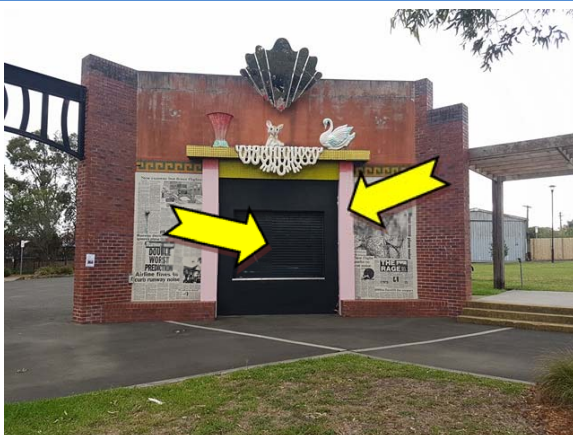
Photo 5. Exterior, south elevation, wall – suspected lead-containing black and pink upper coloured paint systems.
